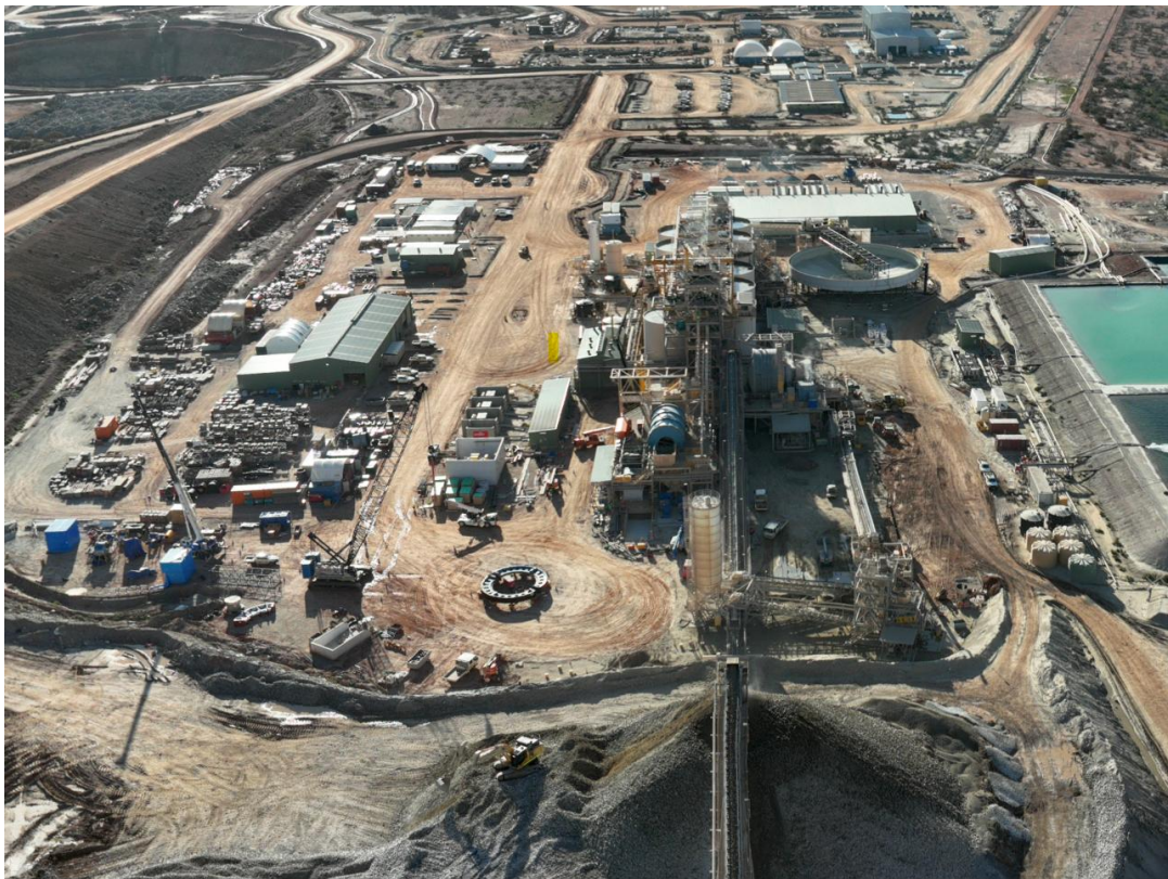
Figure 2: KoTH processing facility
