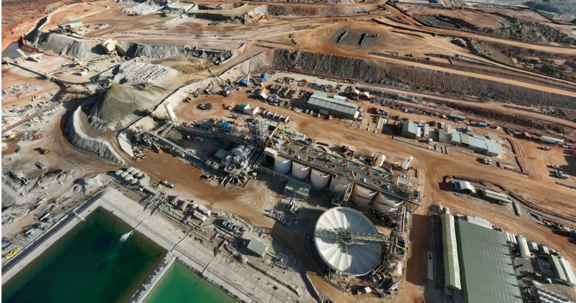
Figure 1: KoTH processing facility
