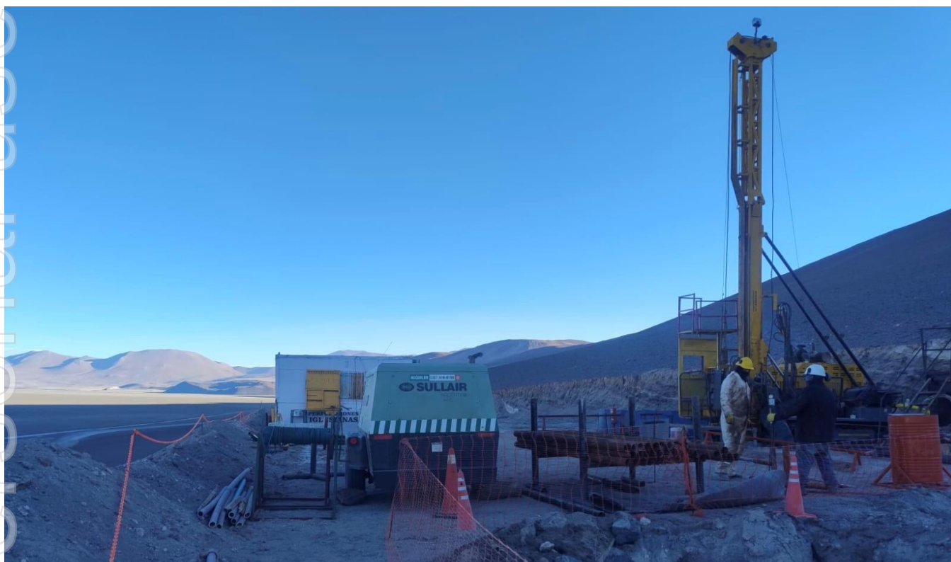
Figure 3 – DDH-3 underway at the Mito tenement
