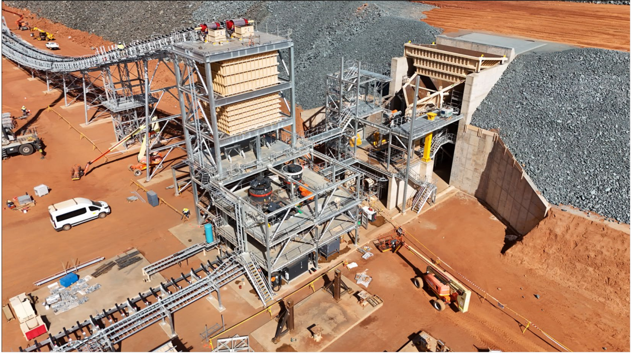
Primary/Secondary/Tertiary crusher building and ROM 2.
