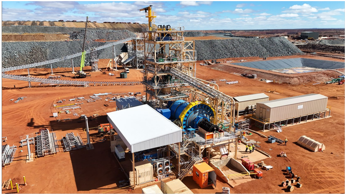
Mill area nearing completion.
