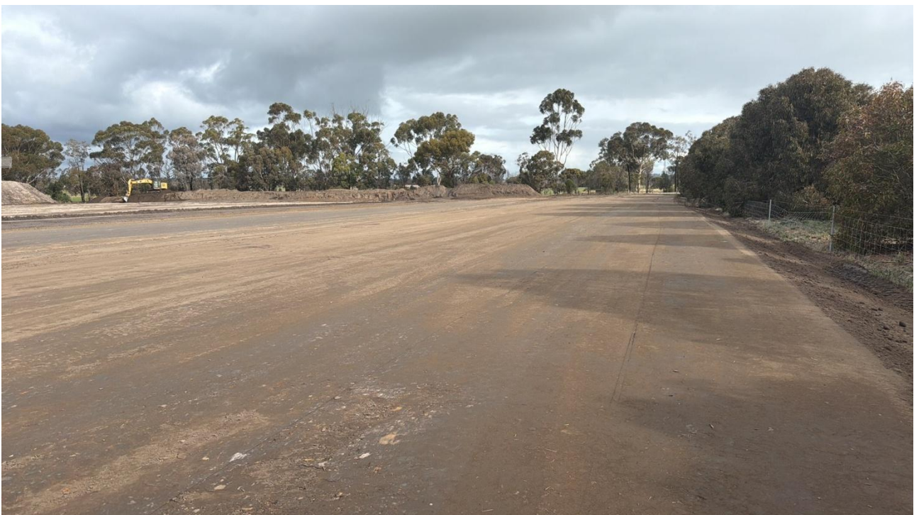
Workforce Accommodation Village site preparation well underway.
