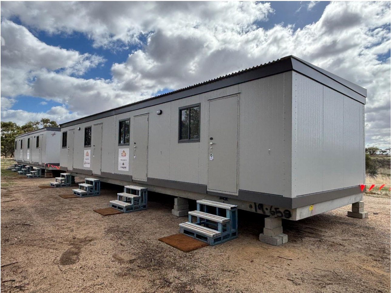
Completed Workforce Accommodation Village modules in Perth awaiting transportation to site.
