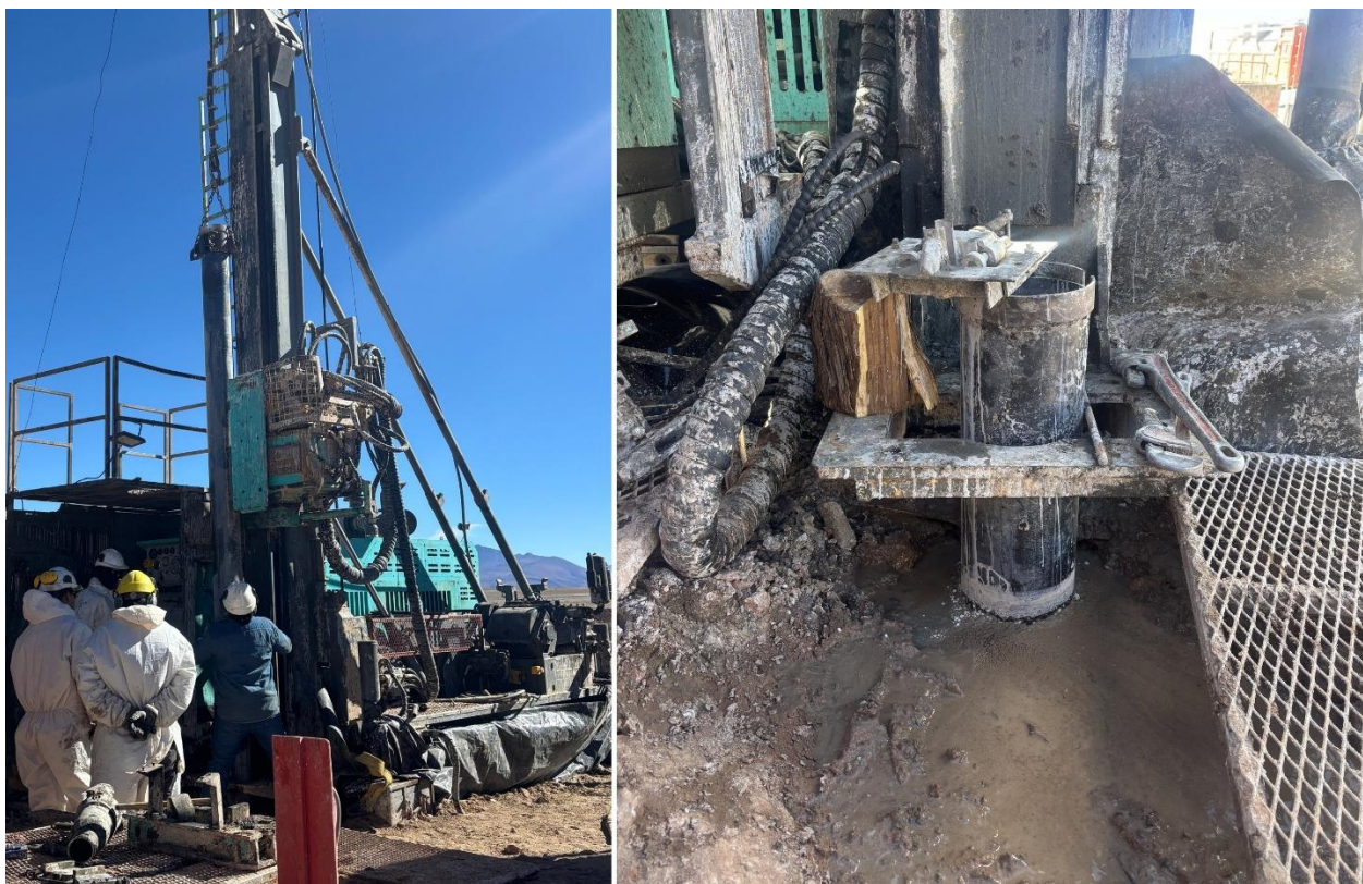
Figure 2. Steel casing going in.
