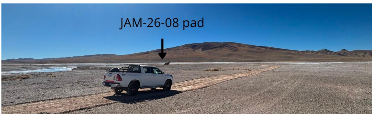
Figure 3. Drill pad location for Well JAM 26-08.
