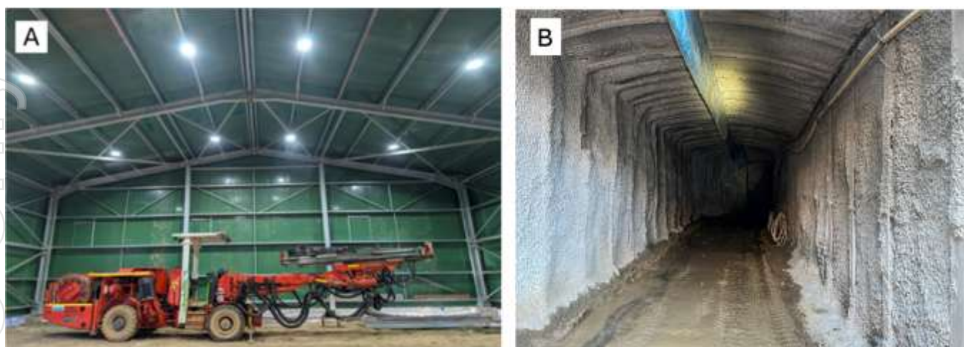
Figure 4 – Photos of the Dittmer mine development. (A) Completed acoustic shed; (B) Portal Shotcreting and Steel Supports.
