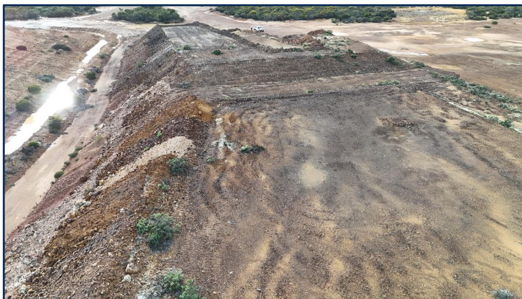
Figure 5: Stockpile at Teddy Bear
