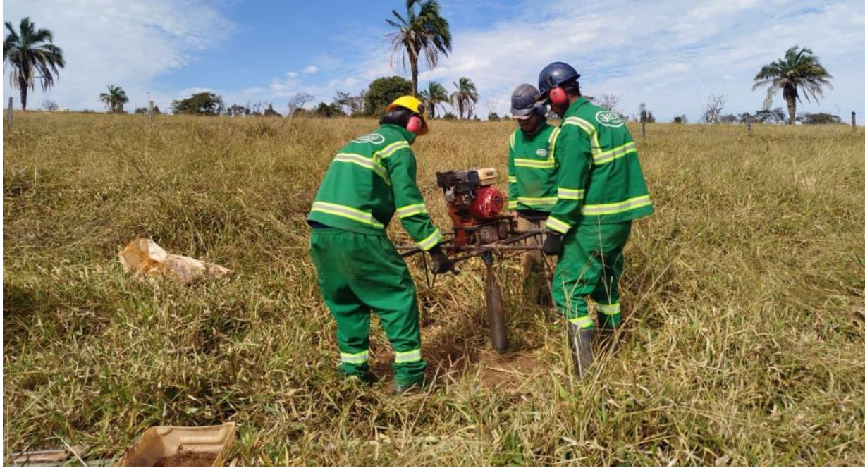
Figure 4: Drilling underway at Piracanjuba. Photo dated 30 June 2026.
