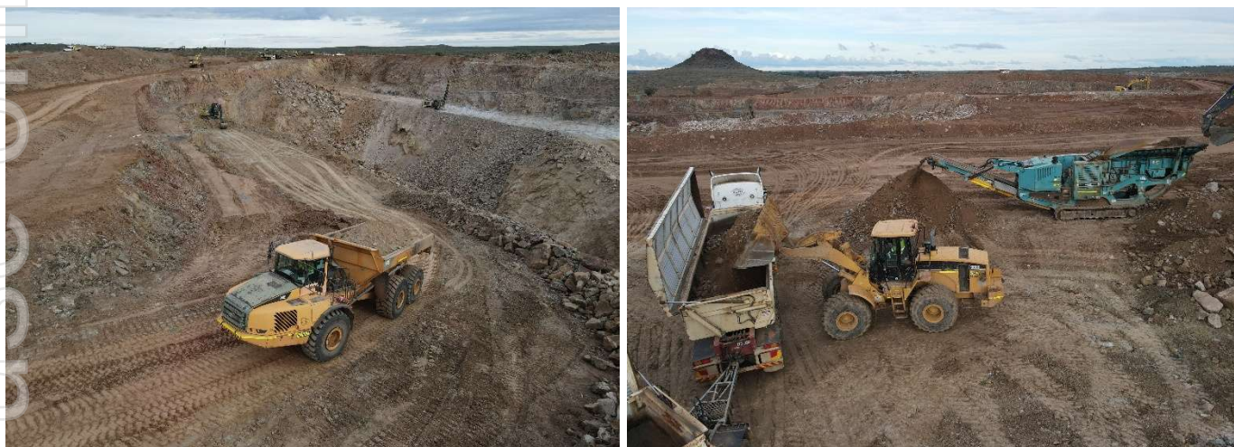
Figures 3 & 4 – Open Pit & ROM operations at the Pinnacles Mine with haul truck loading for transport to Rasp Mill
