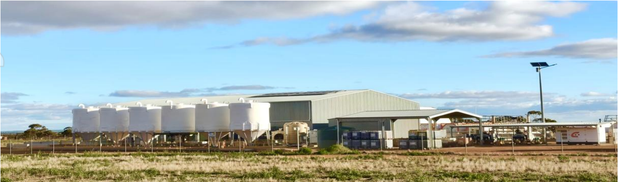
Fig 1. Wubin facility expansion project (June 2026)
