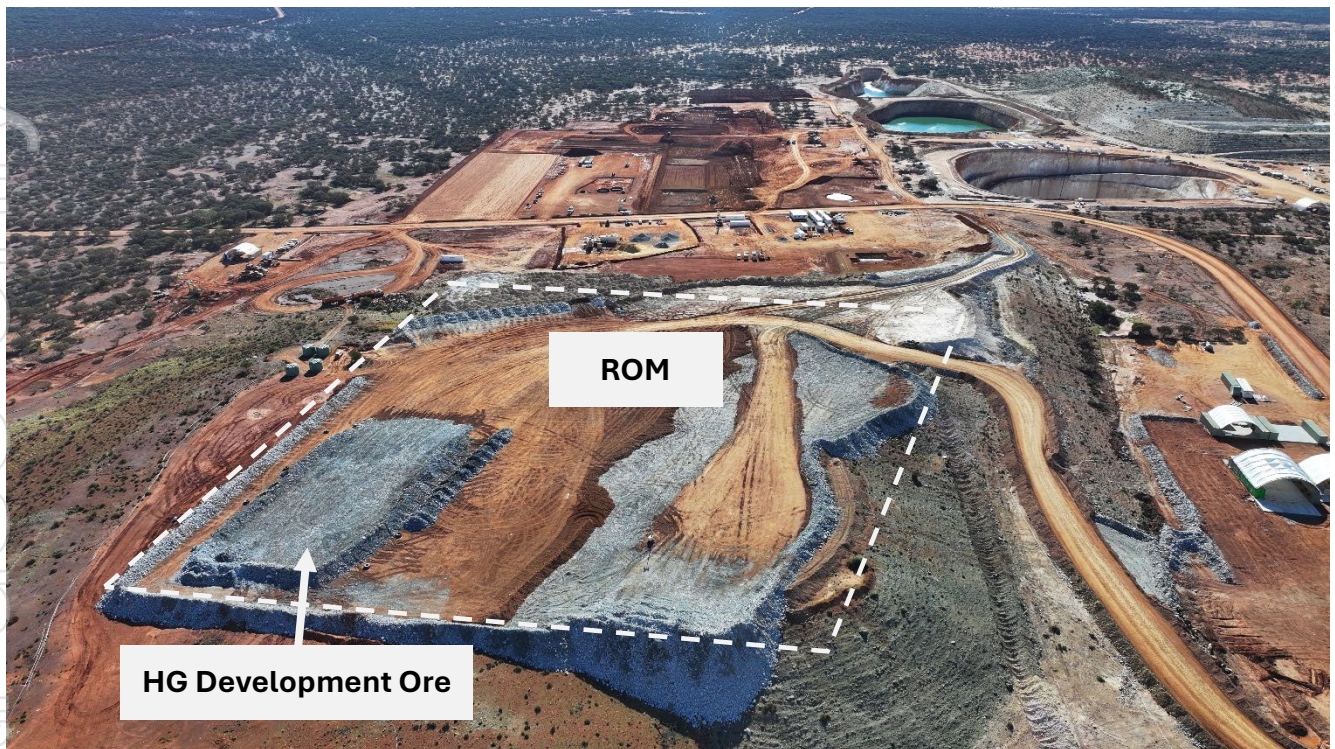
Figure 8 – Ore stockpile build on main ROM
