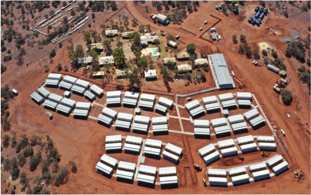
Figure 11 – Camp works nearing completion
