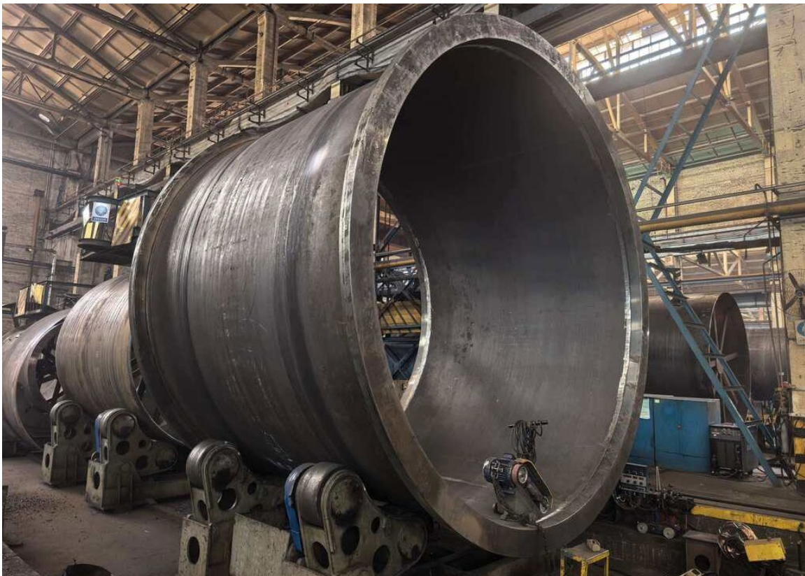
Figure 3 – Ball mill shell fabrication (one of the sections)
