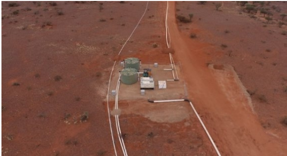
Figure 7: Siphon raw water borefield
