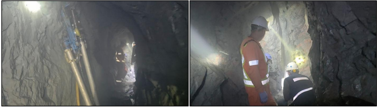
Photos 3 and 4: Development works in the underground levels of Shaft #2 on Santa Barbara Vein #1
