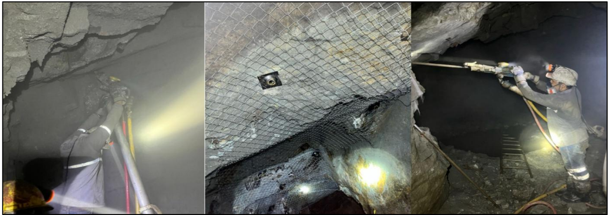
Photos 5, 6 and 7. Shaft 4 ground rock preparation with split sets for ground support
