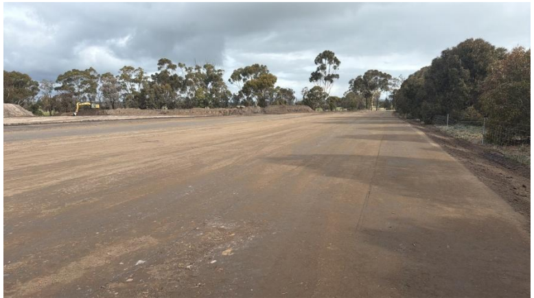
Workforce Accommodation Village site preparation well underway.
