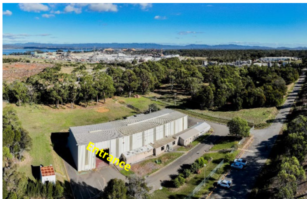
Figure 1: ALCORE Technology Centre, Bell Bay, Tasmania, with Rio Tinto aluminium smelter in background
