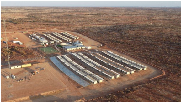
Figure 4: Kurrbili Accommodation Village
