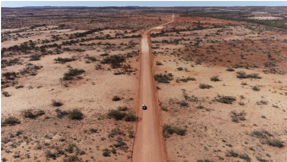
Figure 6: Site access Road Construction
