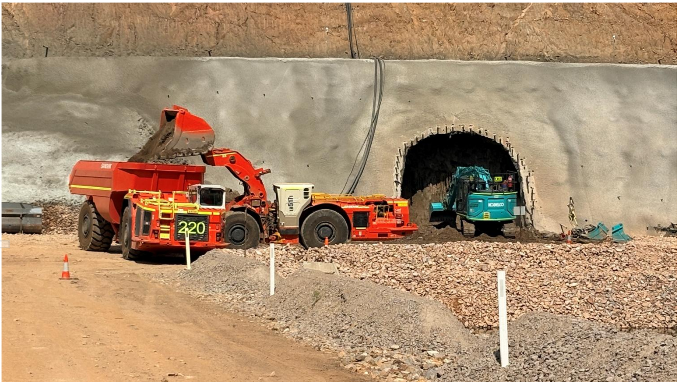
Figure 2 BP33 underground decline progress
