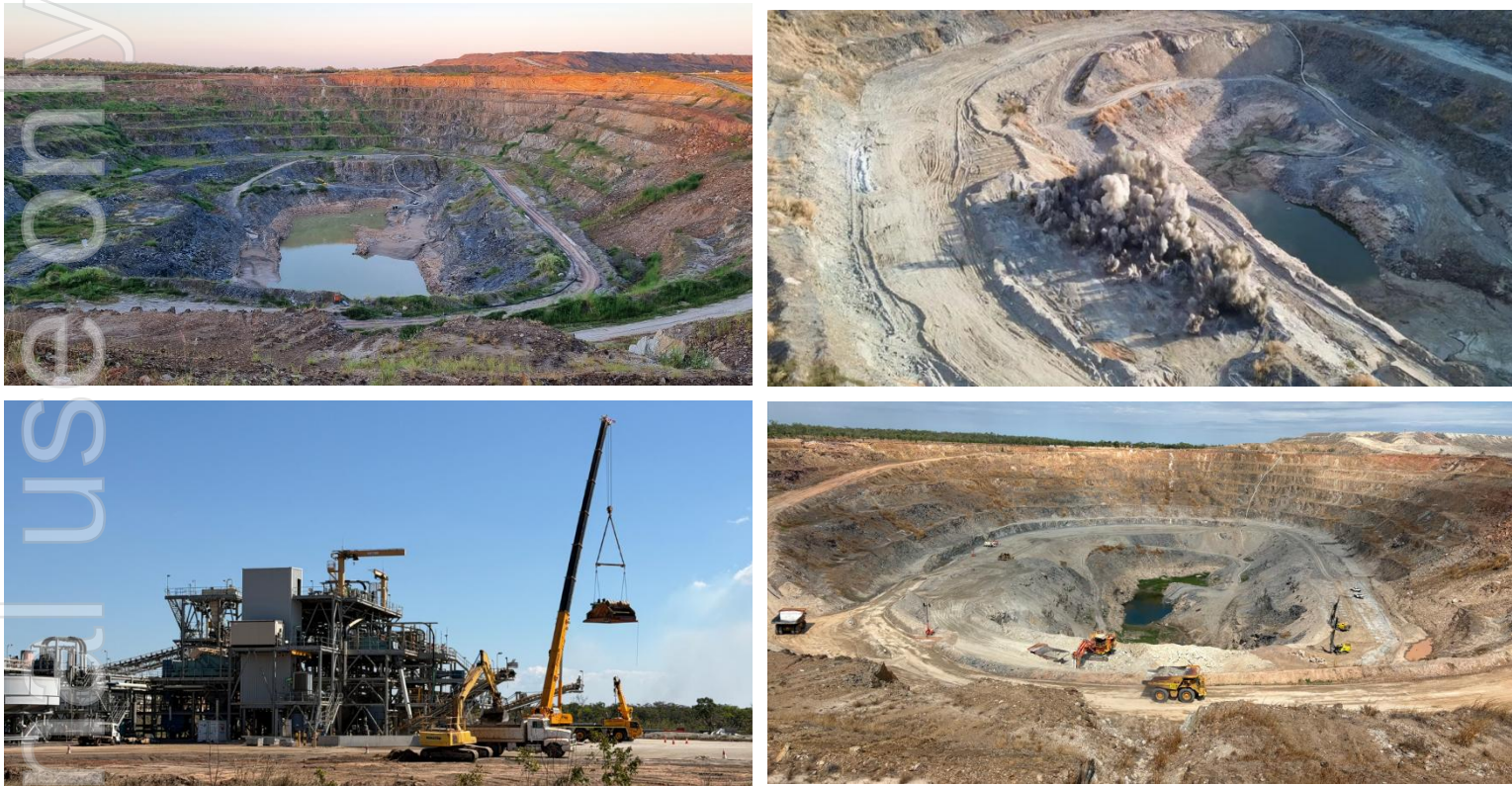
Figure 1 Grants open pit operations (clockwise from top left) 1. Grants open pit April 2026 2. First blast at Grants May 2026 3. Grants open pit June 2026 4. Plant upgrades underway with secondary DMS screen lifted out for refurbishment upgrade
