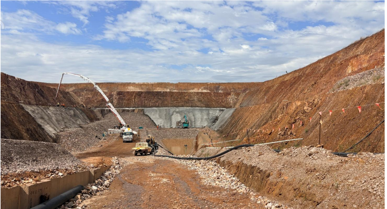
Figure 3 BP33 box cut
