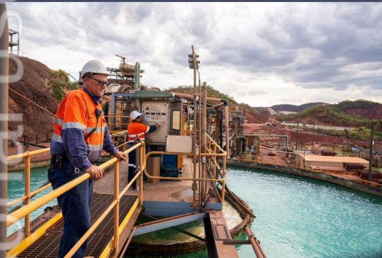
Processing plant & surface infrastructure
