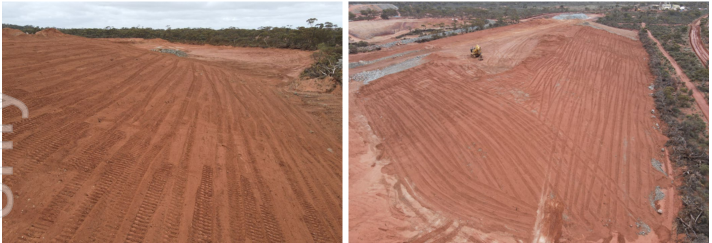
Figure 2: Rehabilitation of the waste dumps continues with deployment of topsoil stockpiles in parallel to the mining operation.
