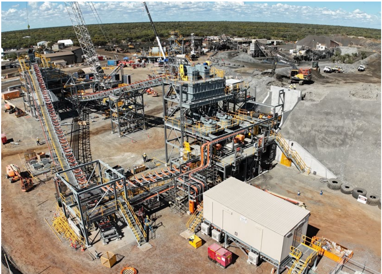
Photo 1: Construction progress - crusher and screening areas.
