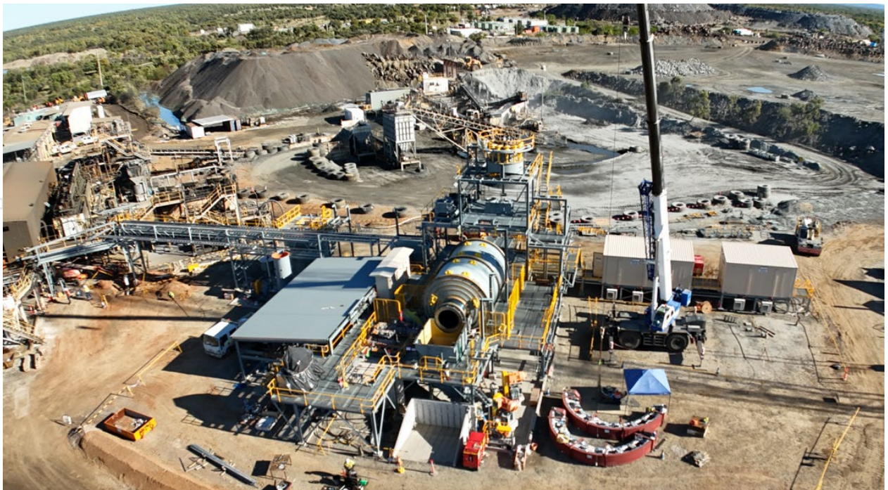
Photo 2: Construction progress – grinding area.
