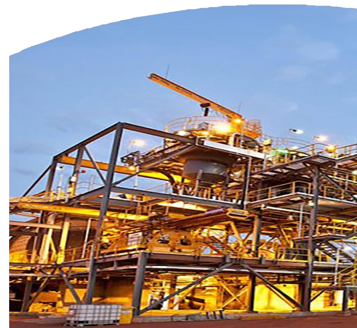
DeGrussa Processing Plant
