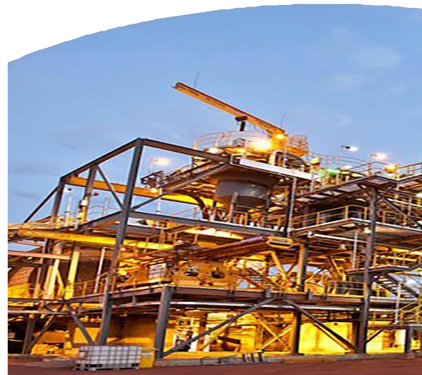
DeGrussa Processing Plant
