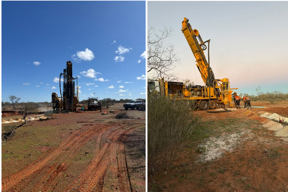
Figure 1: RC Drilling in progress
