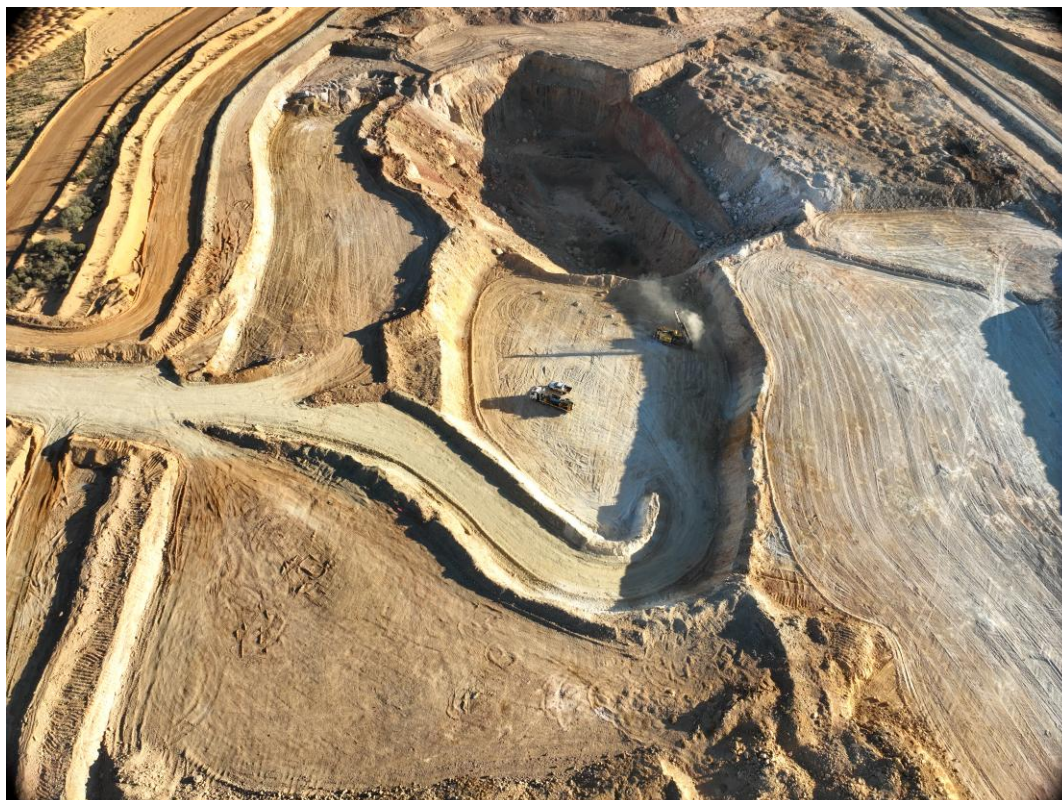
Figure 2: South Pit extension of the Jamaican Rock Pit
