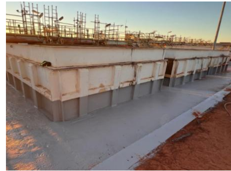
Acid proofing at mixer settlers complete
