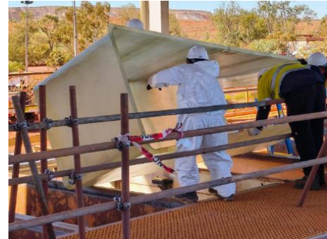
Installing fiberglass inserts for EW cells
