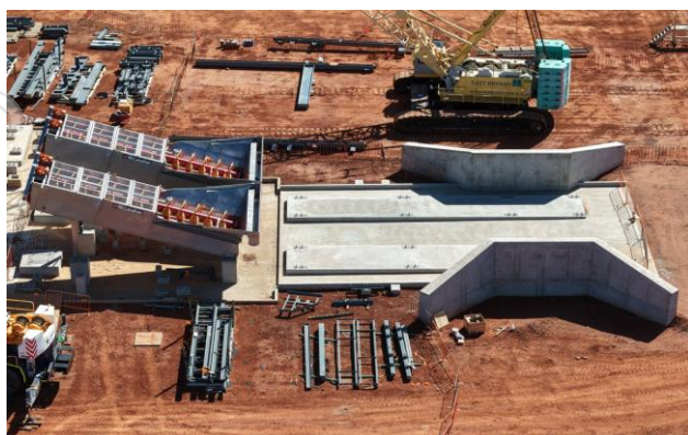
Figure 4: Salt wash plant – Screw classifier installation Figure 5: Crystalliser pond lining and filling
