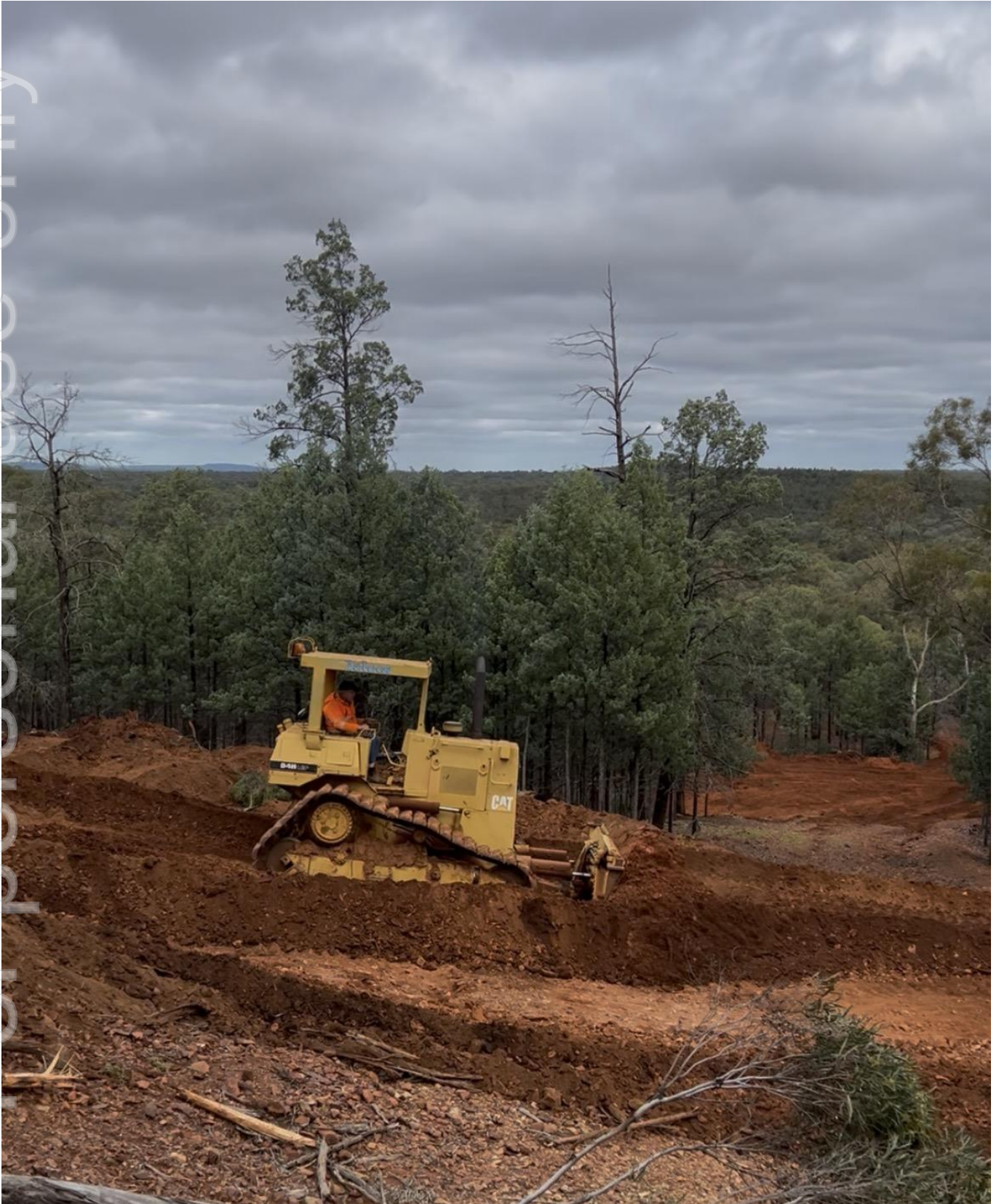
Figure 2: Mt Solitary drill pad/track construction
