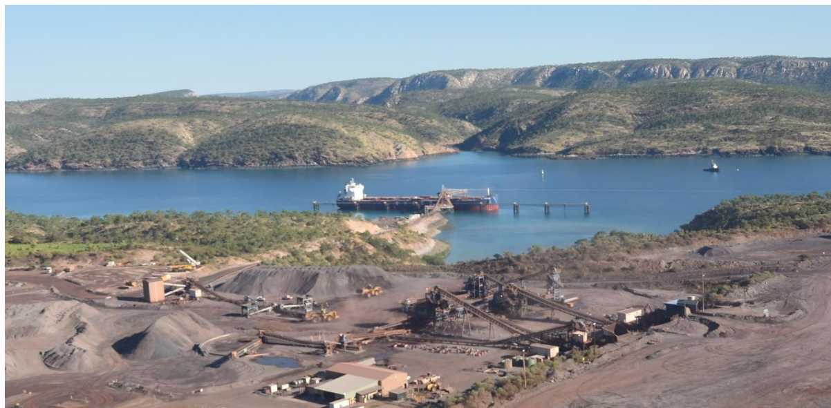
Figure 2 – One of the final low-grade cargoes being loaded at Koolan Island, July 2026.
