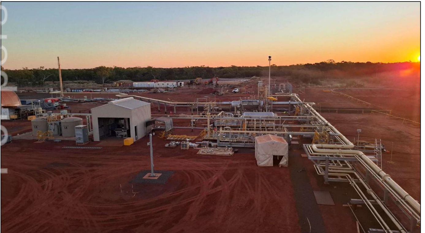
Figure 2: Construction activities of the SPCF
