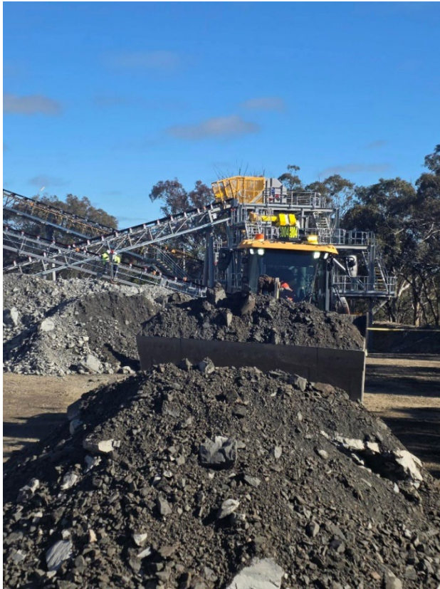
Figure 1 Ore loading on ROM (run of mine) pad
