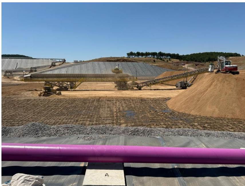
Figure 3: View of the heap-leach pad showing the current status and areas under active irrigation.
