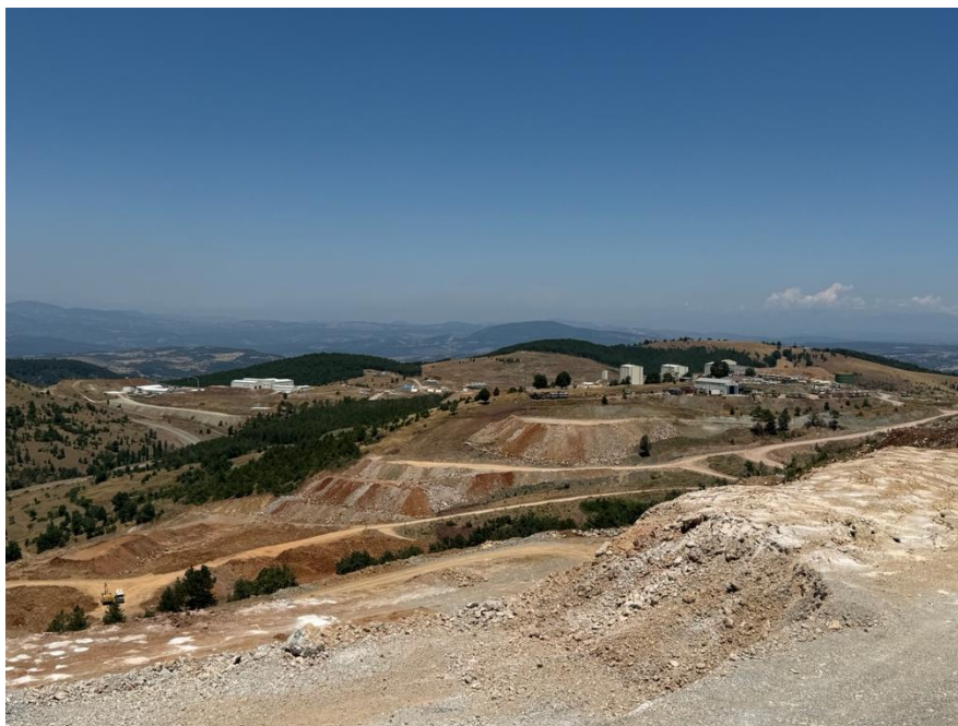
Figure 2: View from the Çakmak Pit (previously North Pit) overlooking lower grade stockpiles, with the crushers and screens buildings to the middle right and mine office and depot facilities to the middle left of the frame.
