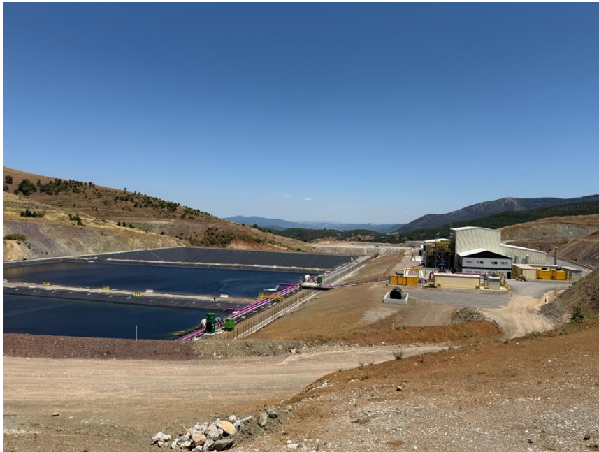
Figure 4: ADR processing plant to the right and the processing water ponds to the left.
