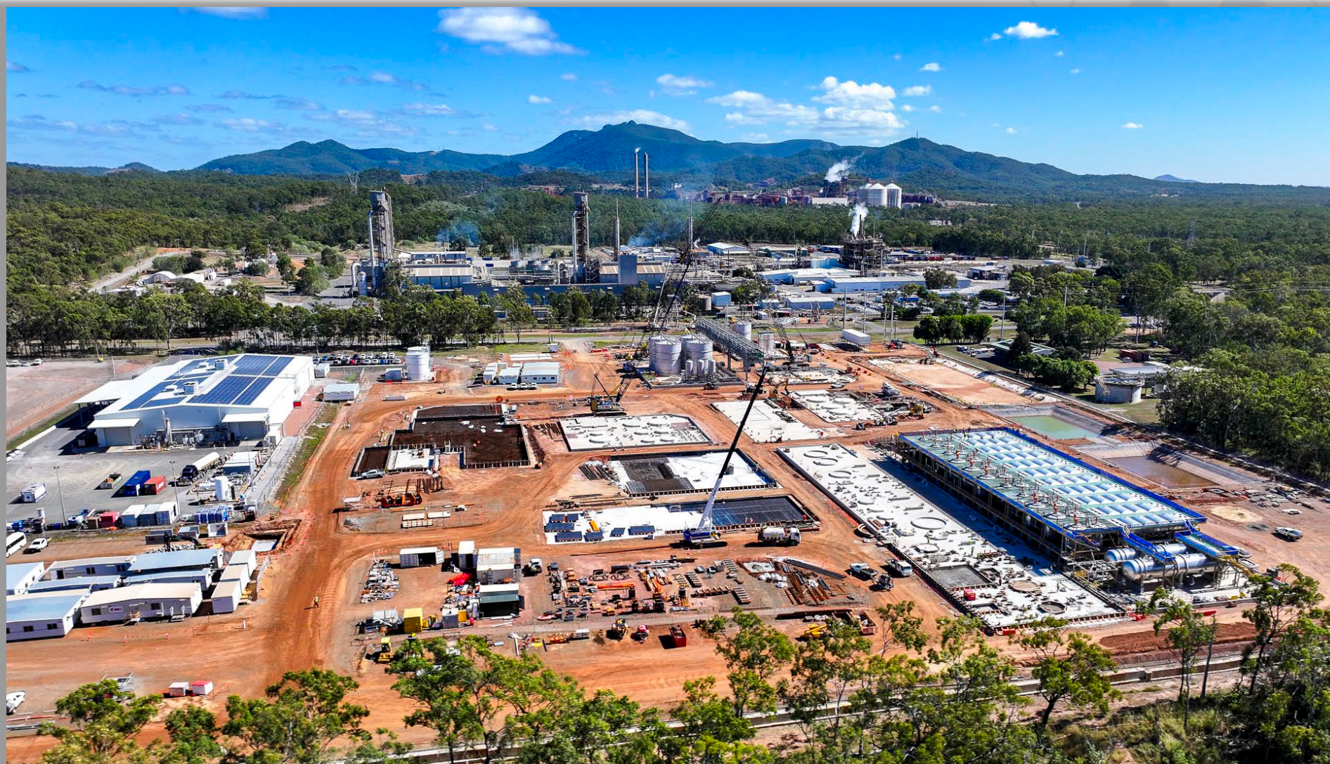
Stage 2 construction – looking west.
