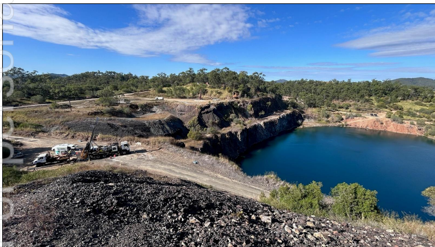
Figure 2 - Rig 2 drilling within the Western Metallurgical Zone.
