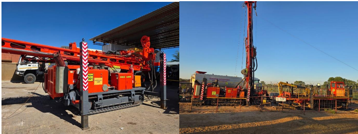
Figure 3 – Rots Drilling rig Mobilised to the KCP
