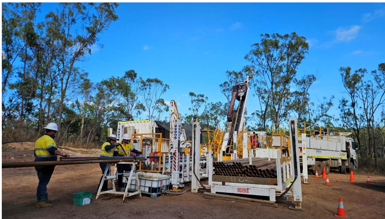
Figure 4. Diamond drill rig at Mt Dillon.
