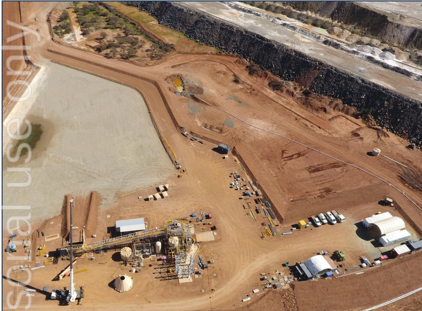
Paste plant construction
