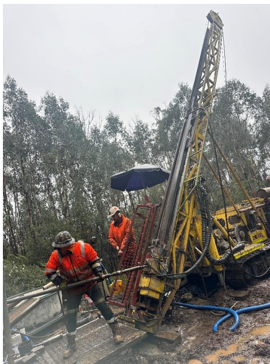
Figure 1: Drilling underway of 26SSDH004
