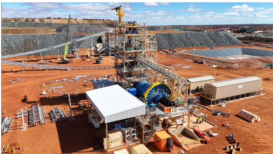
KGP Expansion Project nearing completion July 2026.
