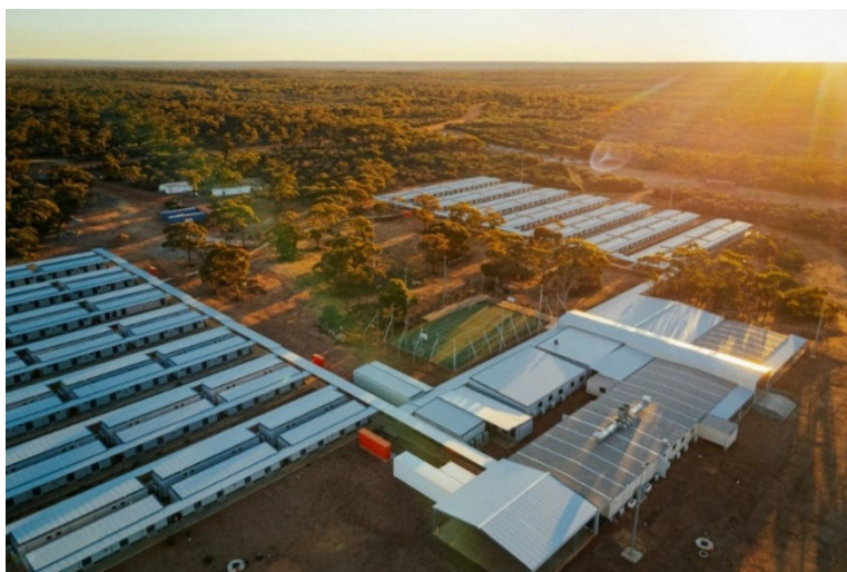
Mount Gibson Gold Project Accommodation.
