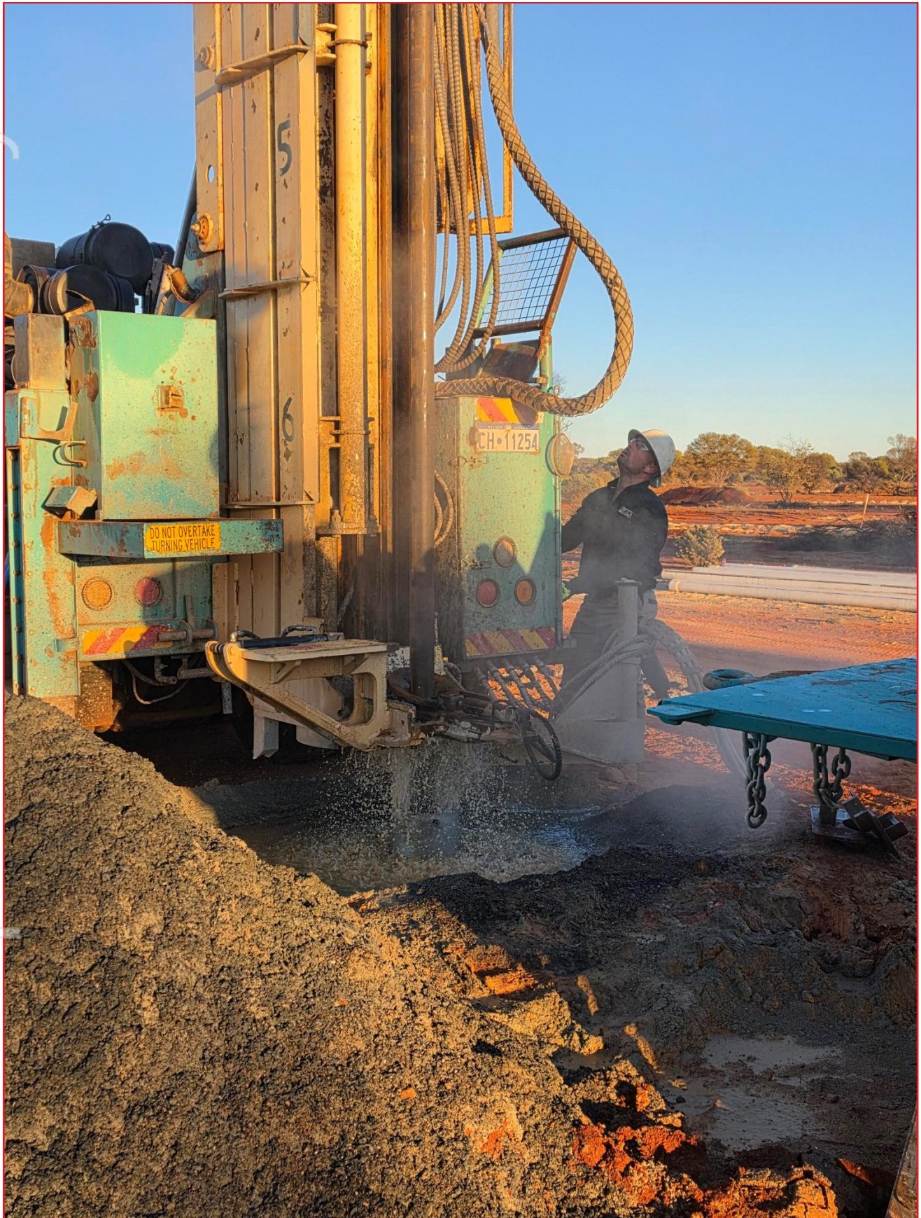
Figure 1: Fresh Water Bore Drilling for the Heap Leach Pad Operations Has Begun
