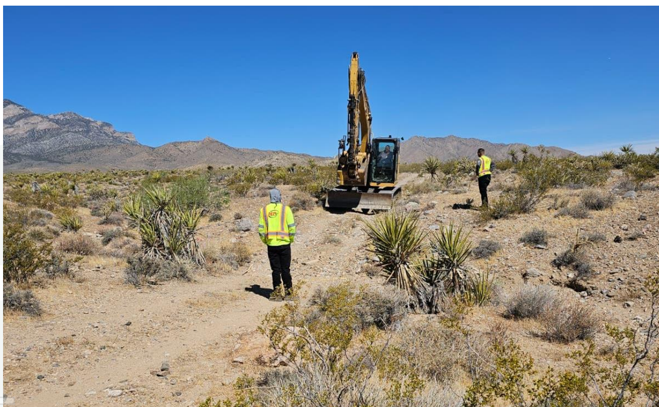
Figure 1: Access track upgrade works at Desert Star
