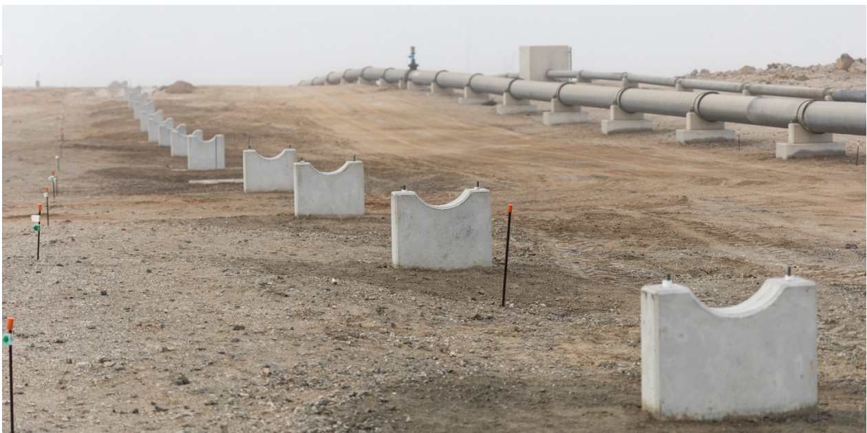
Figure 7: Installation of concrete pedestals for the permanent Etango water pipeline is underway.
