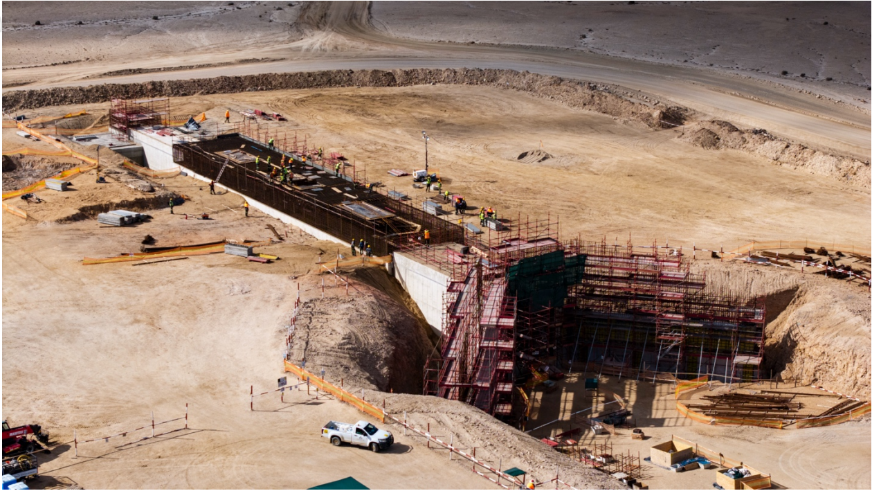
Figure 4: Aerial view of the stockpile tunnel where the concrete roof and wing walls are advancing.
