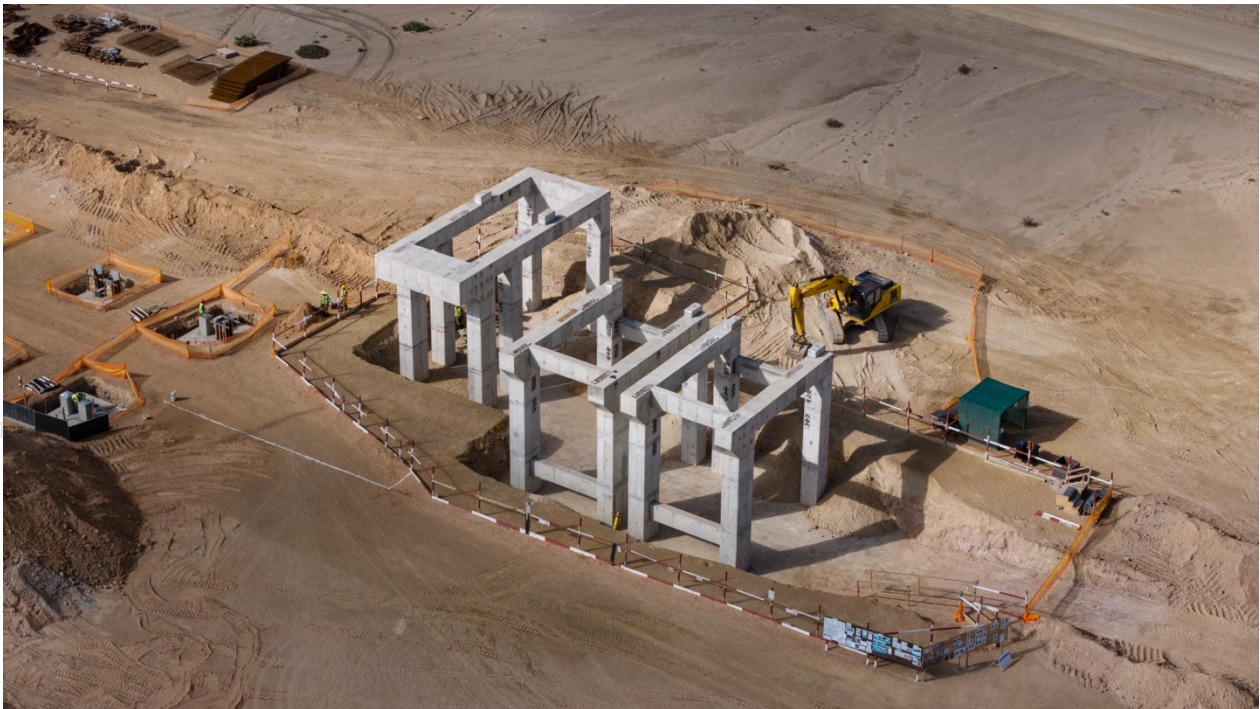
Figure 3: Concrete structures for the secondary and tertiary screening progressing towards completion.
