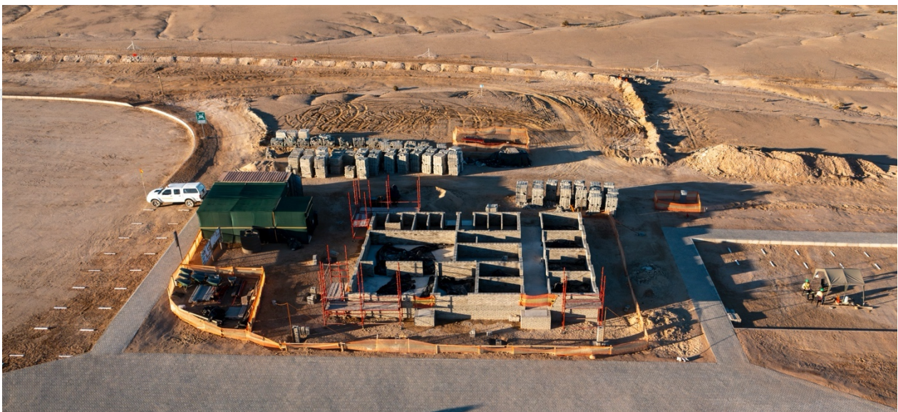
Figure 5: Aerial view of the Etango gate house being built by local Namibian-owned SME contractors.
