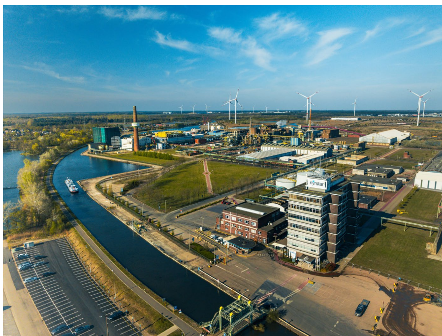
Execution of the A$10.4 million DESALX® project for Nyrstar's Balen site continues.
