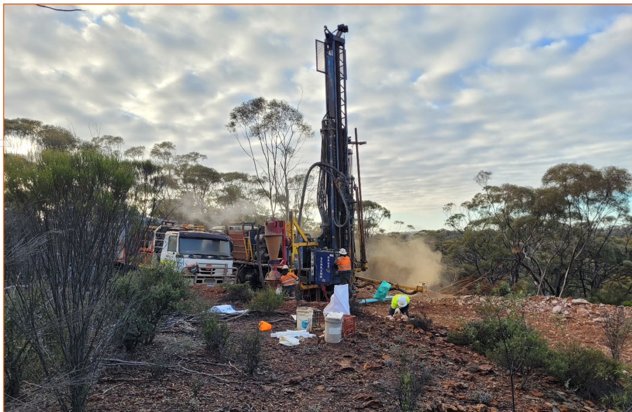
Figure 1: Drilling at Munda - 22 July 2026
