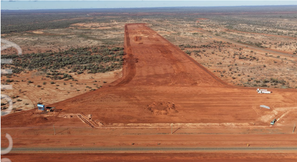
Figure 6. Tower Hill - Construction of new Leonora Rail Terminal underway
