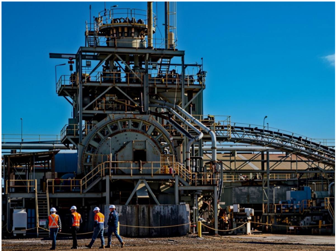
Figure 2: Edna May Processing Facility
