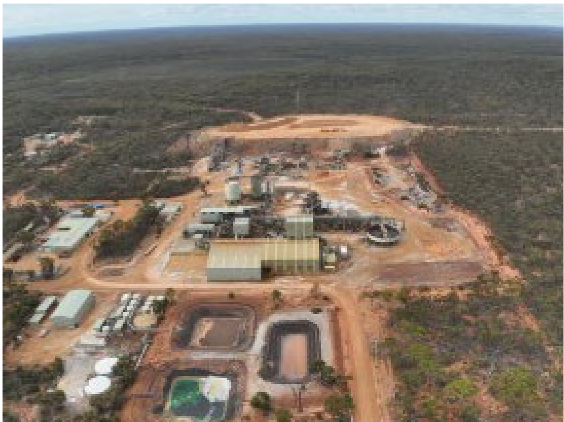
Figure 3: Lake Johnston Processing Facility
