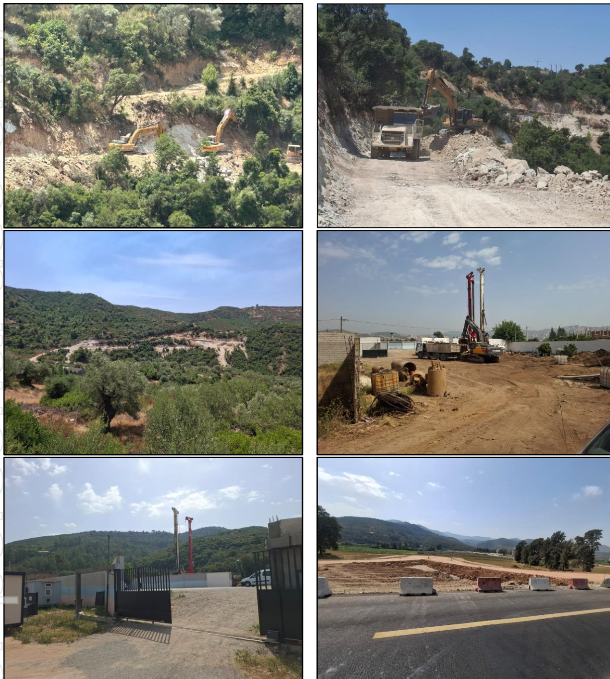
Photos: Activity at the Tala Hamza Zinc, including the construction of the access to the portal, construction of the access bridge and development of the highway interchange.
