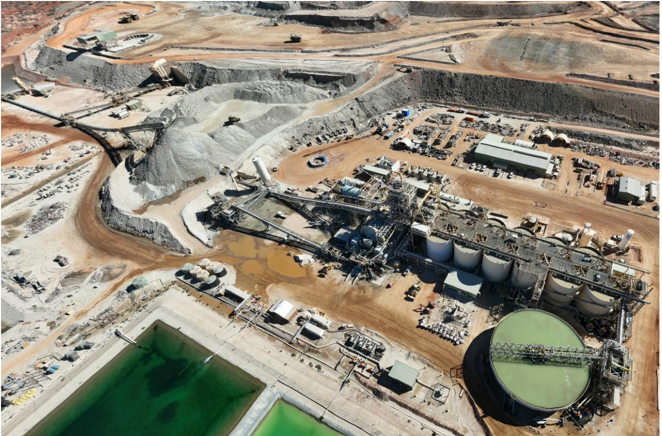
Figure 5: KoTH plant, thickener (bottom right) commissioned
