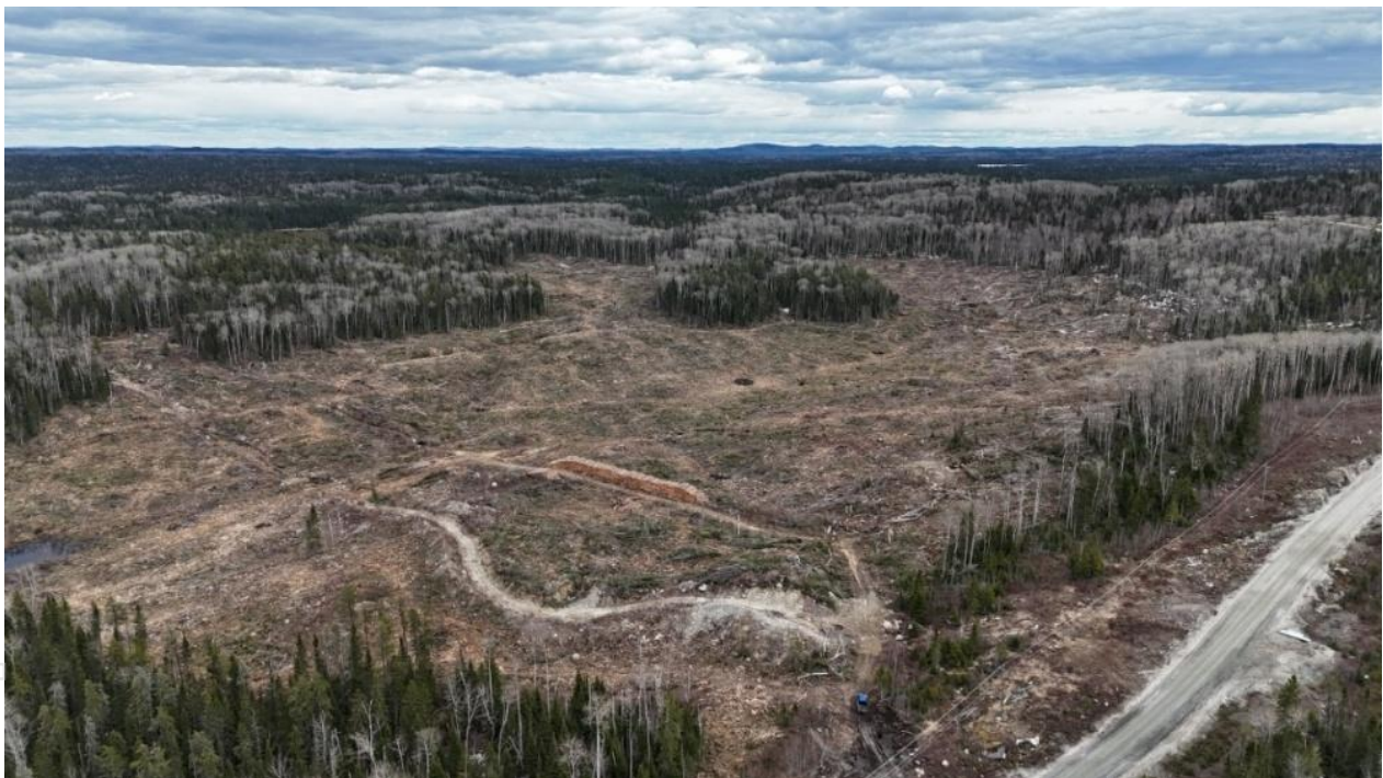
Figure 6: Tree clearing for the STMF completed
