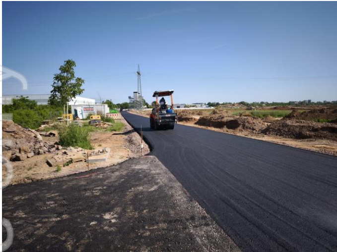
Figure 9: Road resurfacing post ICPP crossing work completion.
