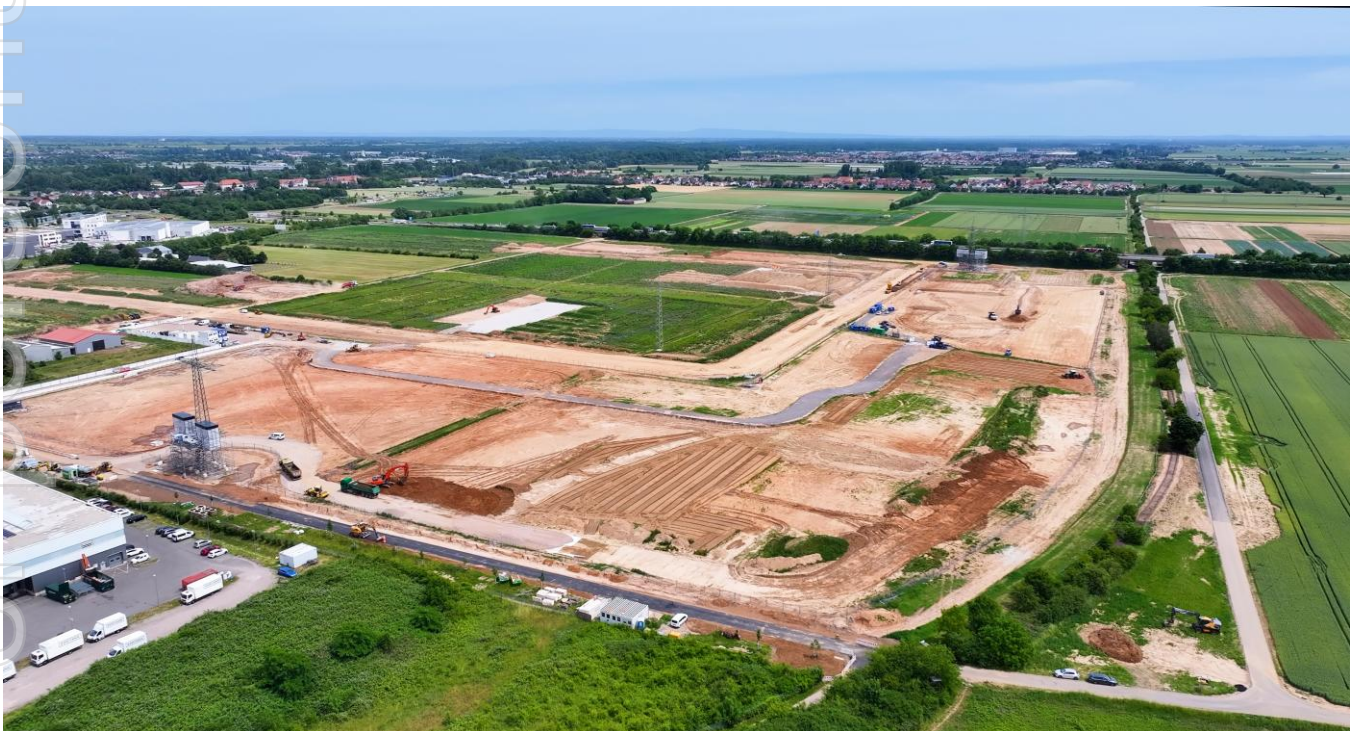
Figure 13: Site preparations at the geothermal and lithium extraction facility in Landau. See overhead powerline infrastructure which is being removed.
