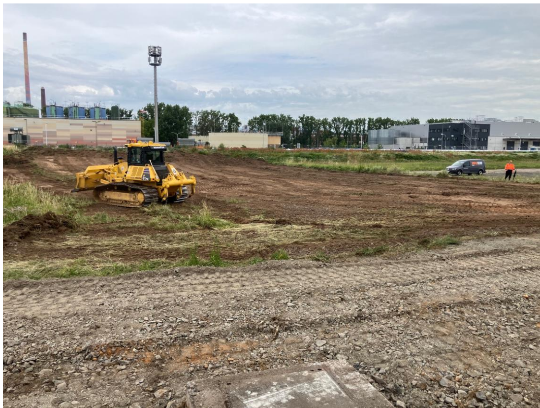
Figure 18: Early bulk earthworks begin at the lithium chemical facility.
