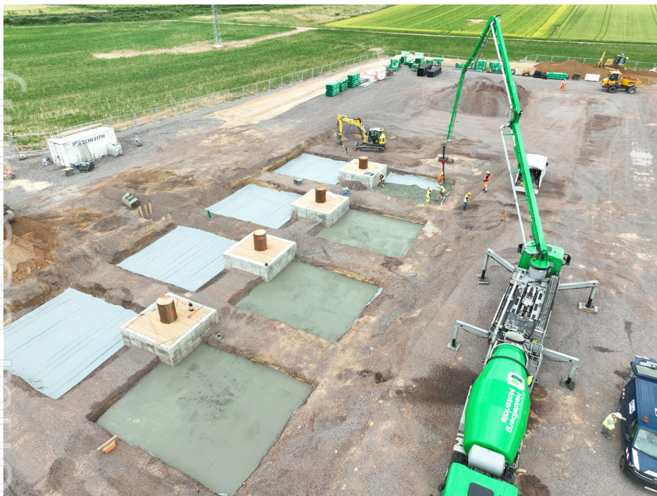
Figure 8: Preparation of drilling cellars at the fourth Lionheart production/ re-injection well site.
