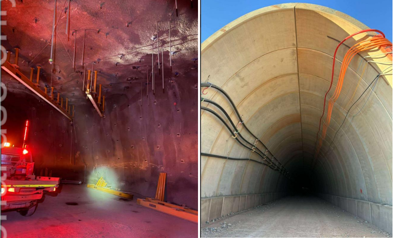
Figure 3: Underground pump station monorail installation (LHS) and completed Main portal (RHS)
