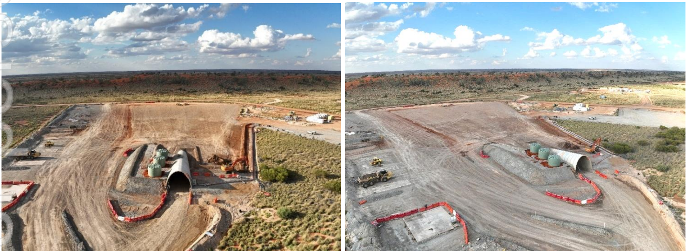
Figure 2: Completed installation of reinforced concrete tunnel and backfilling of boxcut at Havieron portal
