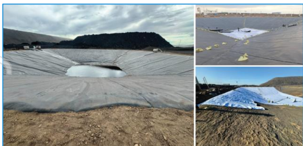
Figure 3 – Pond maintenance completed.
